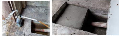
Figure 7. The process of draining the accumulated water around the cubicle ducting
