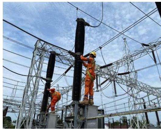
Figure 2. Cleaning process of the bushing
