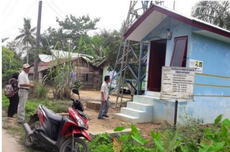
Figure 1. Provision of Clean Water Facilities in Dusun IV Alur Hitam, Securai Selatan Village, Babalan Subdistrict, Langkat Regency
